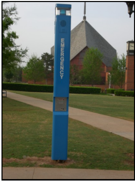
New emergency phone installed as part of the Emergency System
